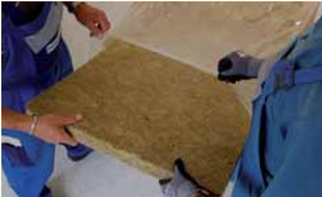
Sliding in the acoustic lining.
