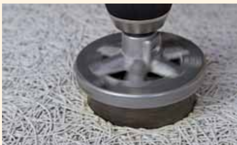
Drilling of a round opening for spotlights, with the exposed surface of the panels up.
