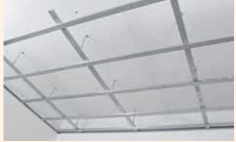
Finished ceiling grid.
