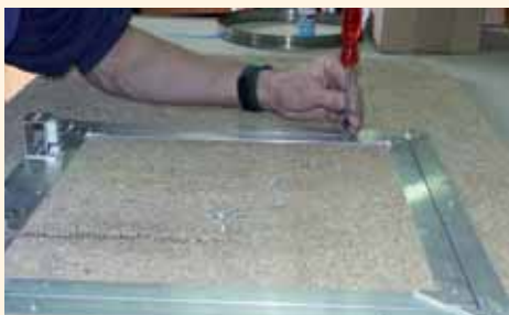
Screwing of the cover plate with at least 2 x 4 screws (4.5 x 20 mm) per frame (40 x 40 cm) or 2 x 6 screws for 60 x 40 cm and Heraklith-BM PU or polymer glue on the inner frame.
