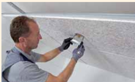
Insertion of the housing of a spotlight.
