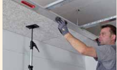
Align the panel rows with an installation lath. Panel joints must be positioned to be centred under the section. No free, suspended panel joints are allowed. When installing square panels, observe the installation direction marked on the back of the panels.
