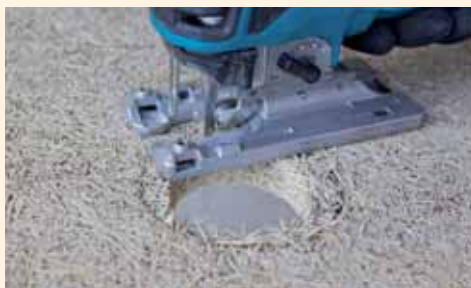
Cutting out an opening with a jigsaw, with the exposed surface of the panels down.
