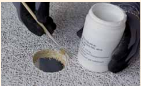
Cover cut edges with paint if these are not concealed by a cover.
