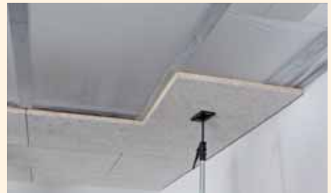
Alternative: insertion of PE sheet as trickle protection or a vapour barrier matching the installation of the Heradesign acoustic panels. Gluesheet joints together.
