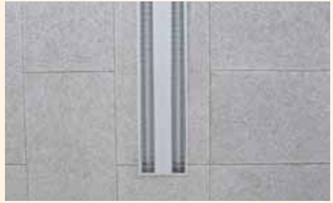
Installation of a grid light. Two additional load-bearing sections have to be installed. Disengage basic sections and place additional hangers.
