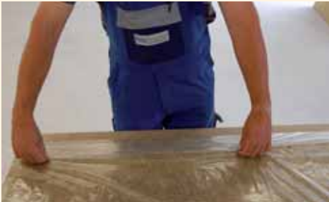
Folding over the film edges.
