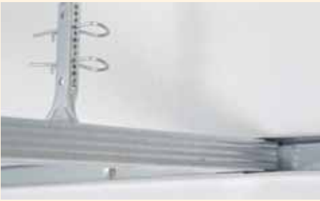
Wall connection of the CD-sections with UD-28/27 wall connection sections as an alternative to E wall connection sections.
