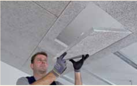
Installation of a maintenance opening. The load-bearing section must be disengaged.
