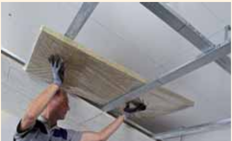
Insertion of KI mineral wool piece by piece along with the installation of the Heradesign acoustic panels. Absorber panels that are jammed between the sections are cut to size. For EI 30 structures, the first layer of rock wool panels is placed on the load-bearing sections, the second layer on the basic sections. Joints must be tight.
