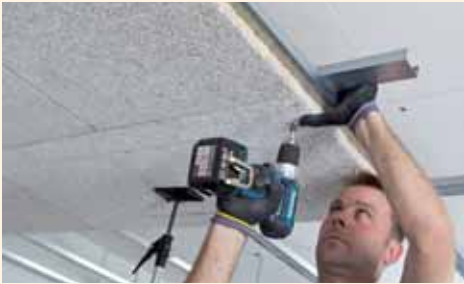
Install the acoustic panels by means of supports. Press the panel onto the section with the ball of your hand while screwing. There must not be a gap between the acoustic panel and the section. Start panel installation from the centre of the room. Only work with the acoustic panels with clean hands and clean tools.
