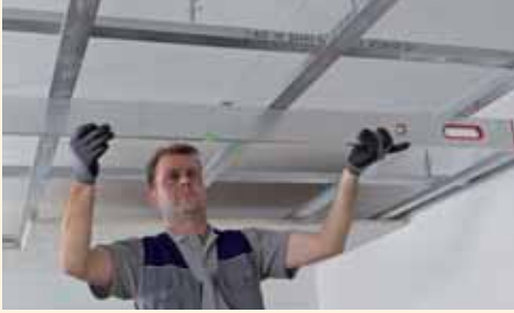
Aligning the CD-sections with a spirit level or laser level.
