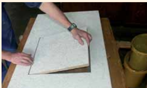
Insertion of the cover plate.
