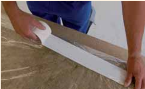
Taping up the film end.
