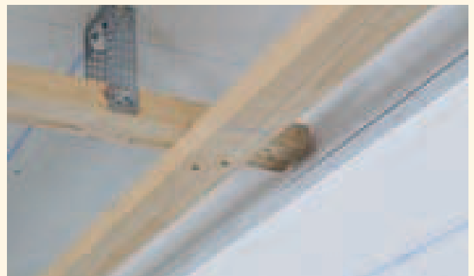
Maximum spacing of main and cross joists to the wall, see sketch on page 4.
